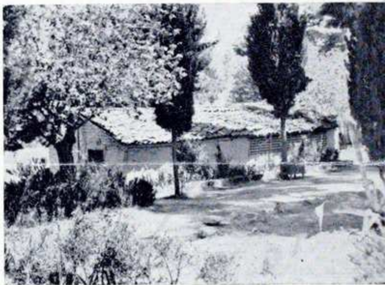
Buildings like this must be replaced
