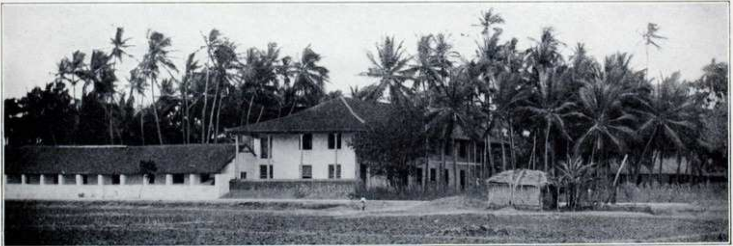
Jaffna College Buildings from the southeast, Jaffna, Ceylon
