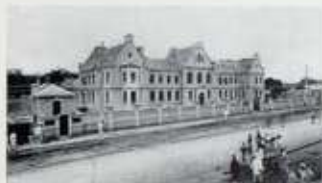
The South China Union Medical College. Buildings owned by London Missionary Society
