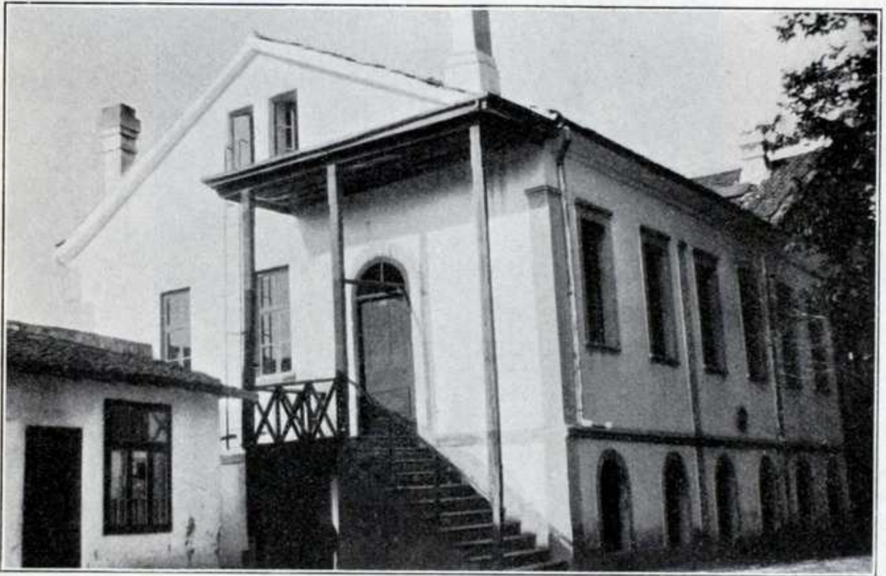
Assembly Hall with Dining Room over.
