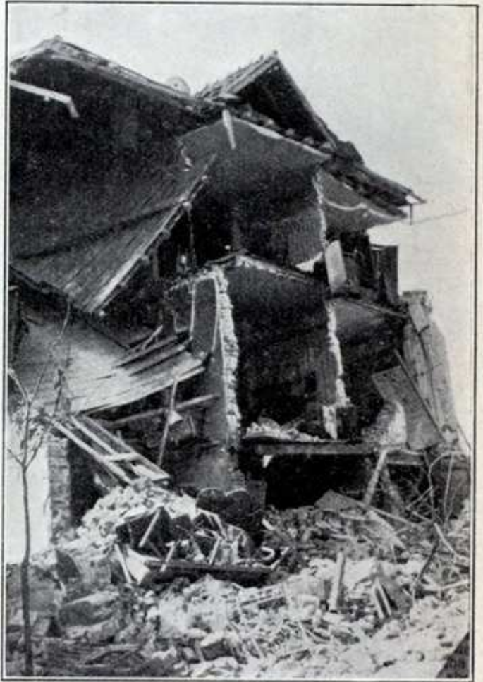
A Ruined Dwelling House, Philippopolis.
